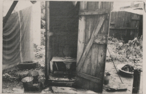
Sanitary system --- laundry, toilet, and water supply.
