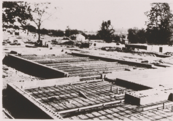
FIRST FLOOR REINFORCING ILLUS. NO. 24.
