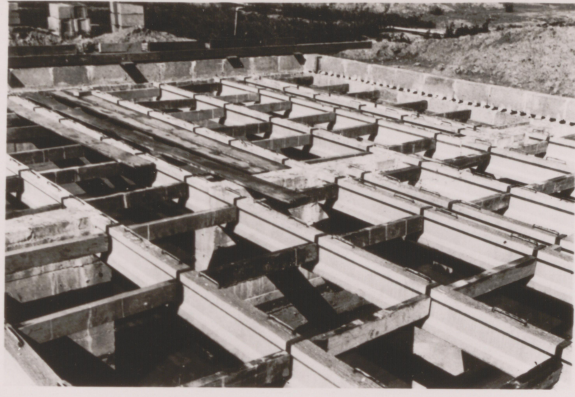
PRECAST JOISTS ILLUS. NO. 23.
