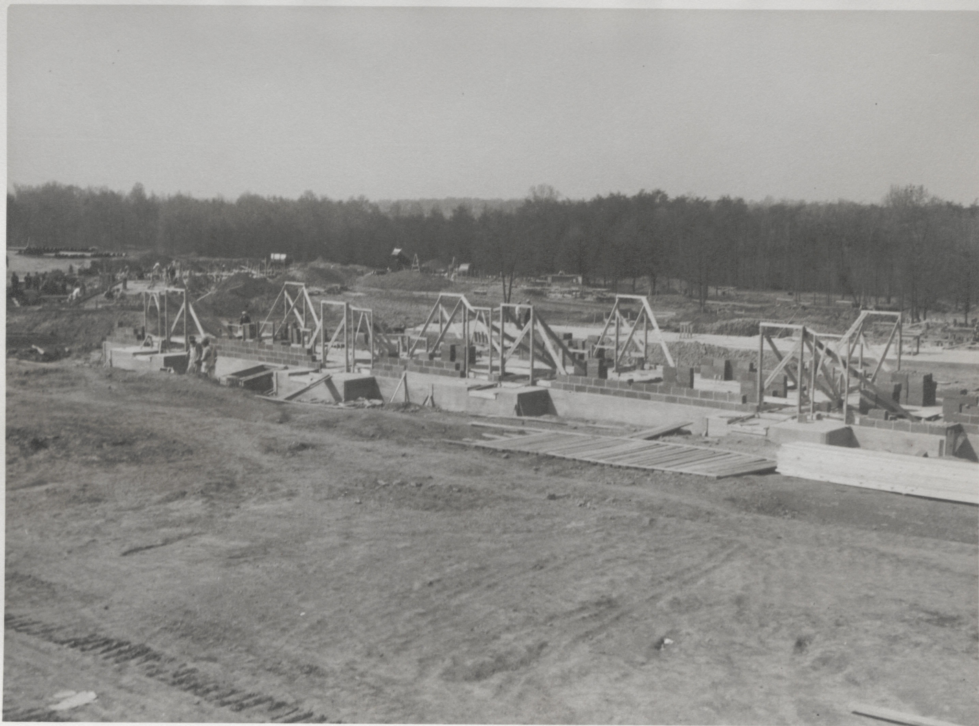
21. CINDER BLOCK CONSTRUCTION STARTED
