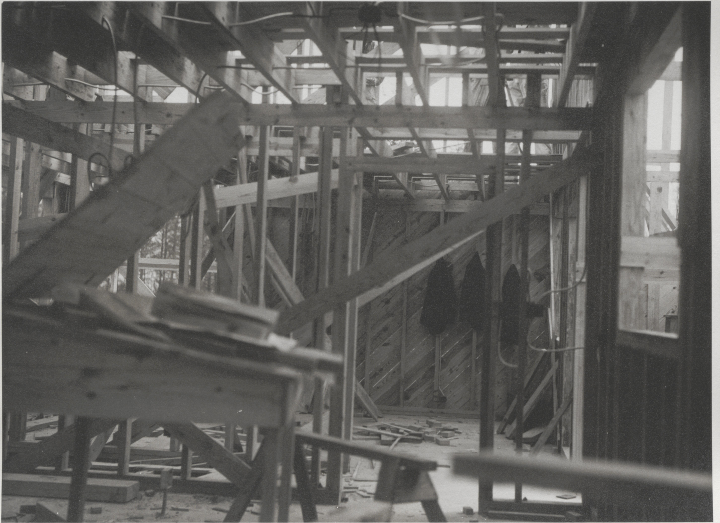
20. INTERIOR PARTITIONS SHOWING INTERIOR WIRING
