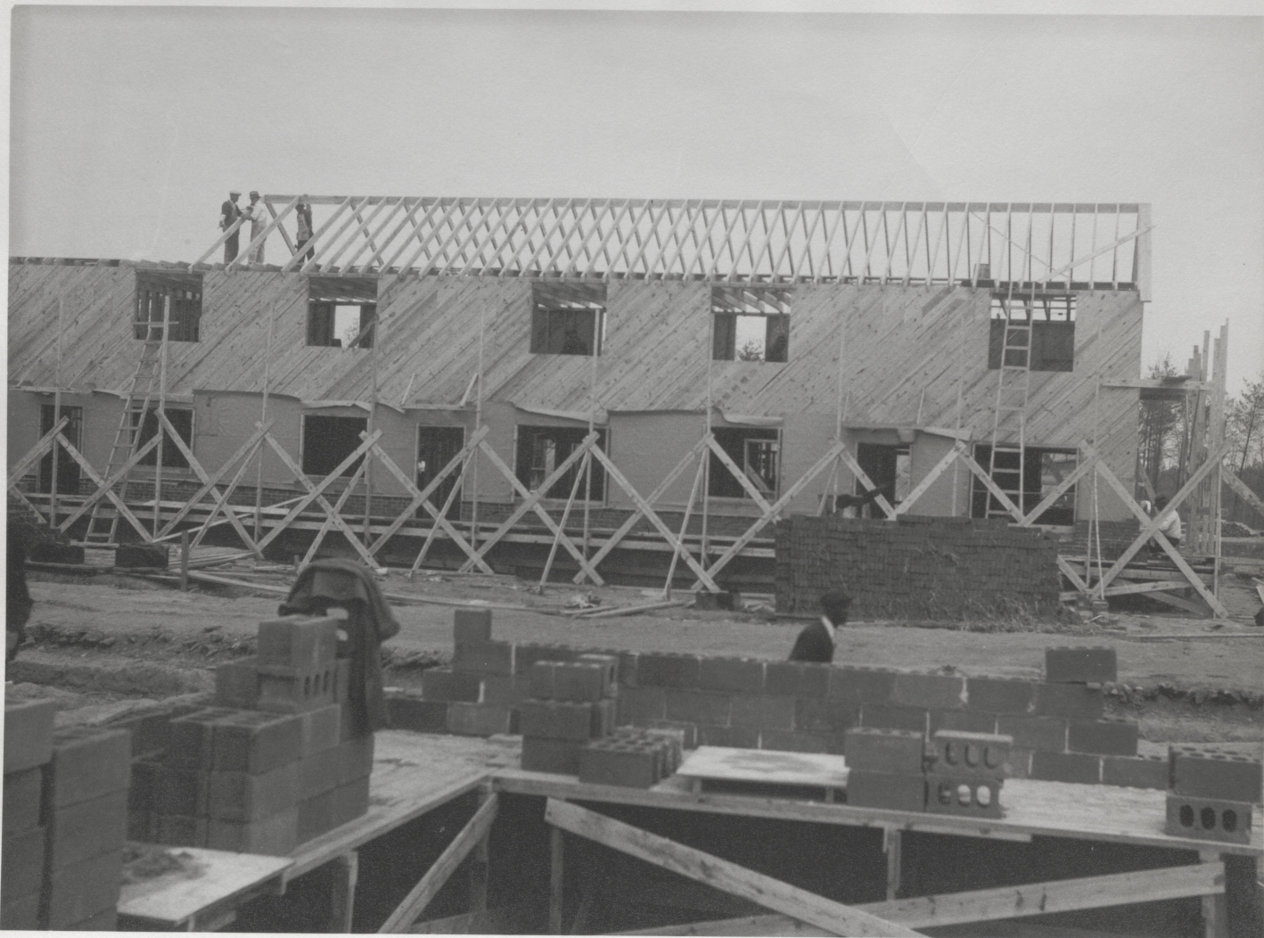
17. FRAMING - ROOF RAFTERS FRAMED
