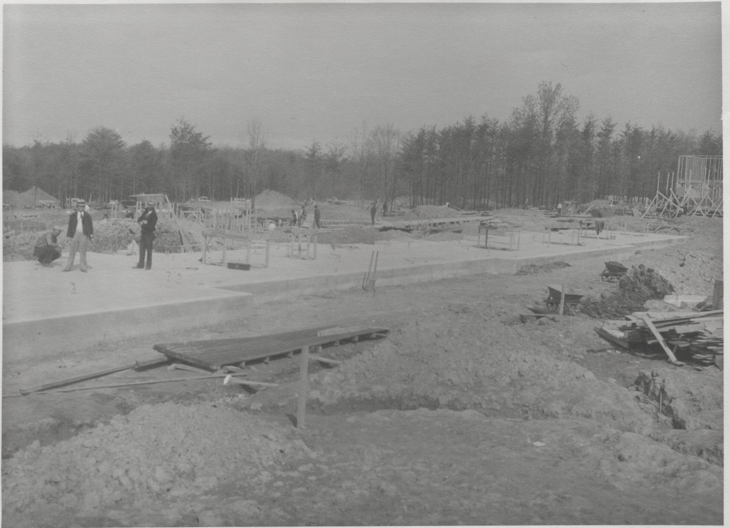
13. FIRST FLOOR SLAB POURED
