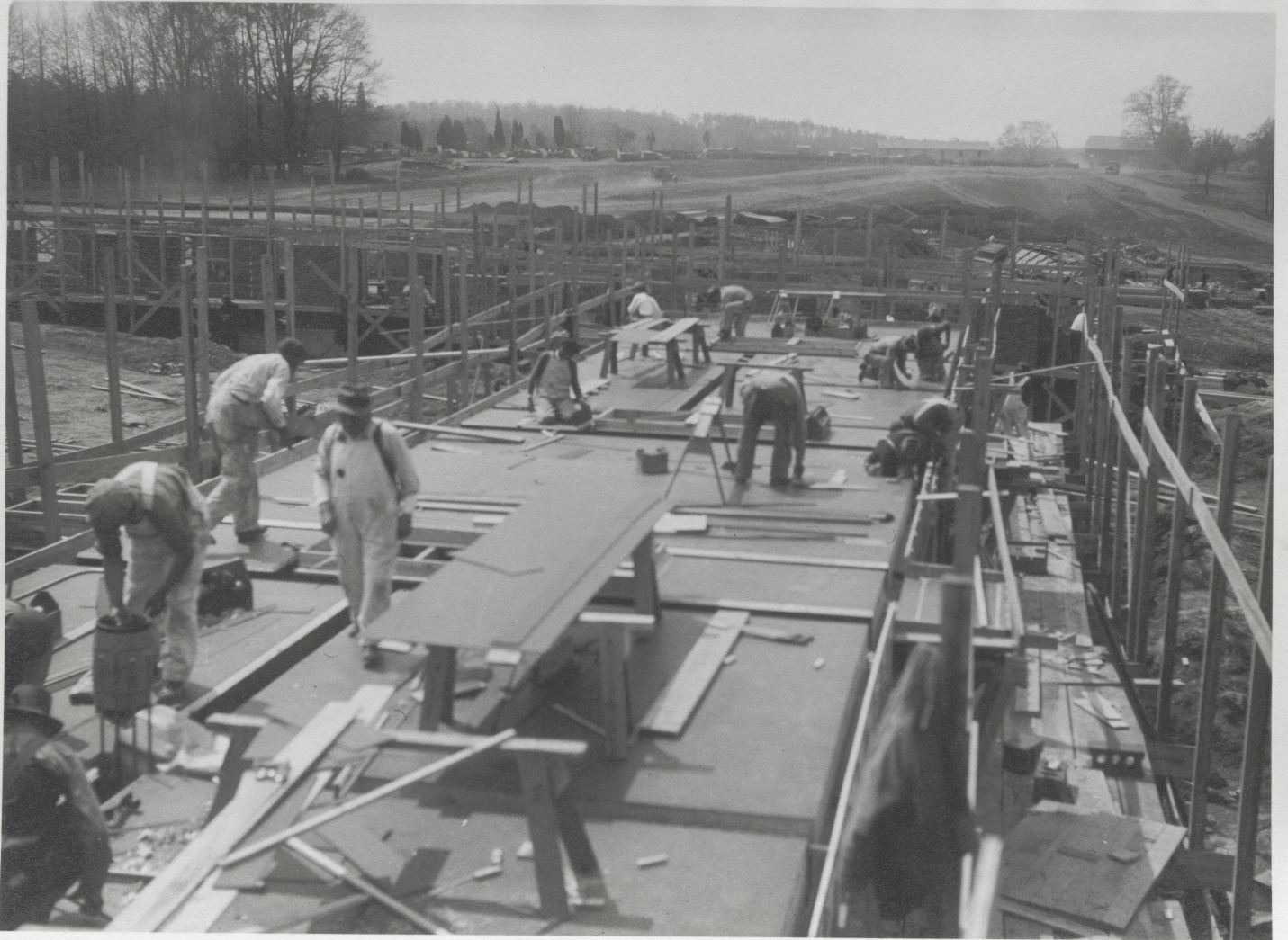
11. FIRST FLOOR SLAB FORMS STARTED
