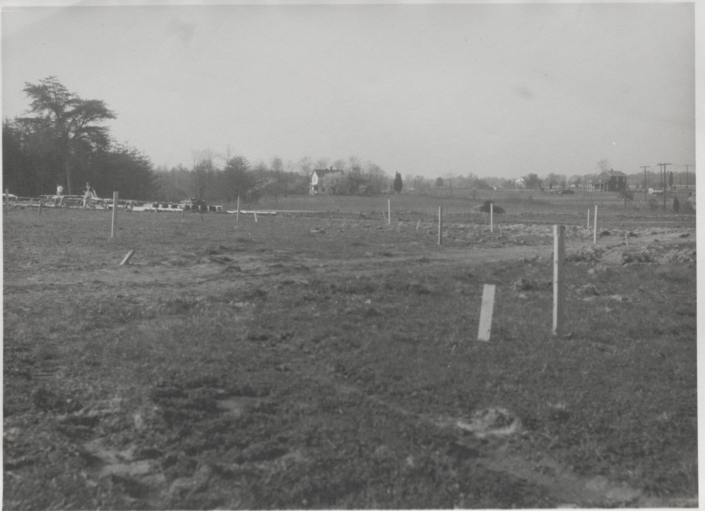
1. SITE STAKED OUT READY FOR EXCAVATION
