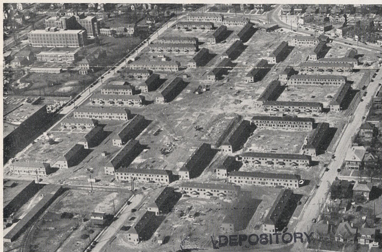
Aerial view taken during construction of Lamar Terrace, recently opened 108-unit project in Memphis, Tenn.
