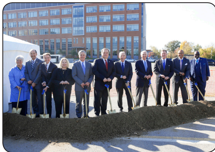
In October President Capilouto, joined by state and university leaders, broke ground on a new research building.
