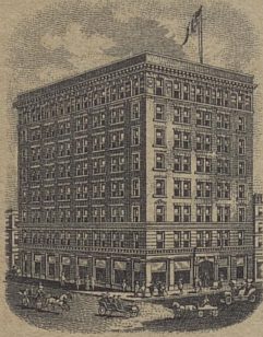
TRUST COMPANY BUILDING.
