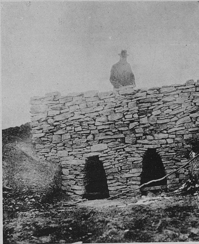
Fig. 2. Front view of a limekiln.
